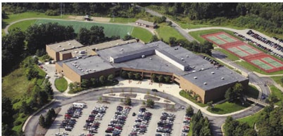
A fully adhered EPDM roofing system installed on Shaler High School in Pittsburgh, Penn., utilized a 60-mil membrane to provide the durability and system longevity required by project specifications.
